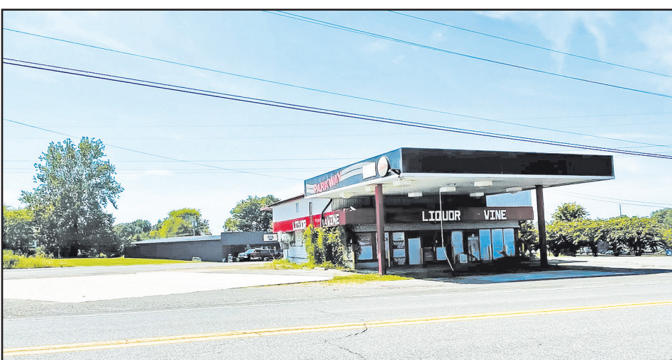
US 51 IMPROVEMENT PROJECT- Plans are for this building on Hwy. 51 S to come down and that area be made into a wide turning area onto Kimbro Street. (Photo by Gaye Bencini)
