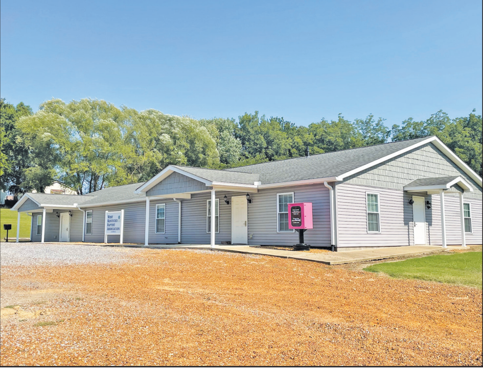
The Hickman County Senior Citizens activities will be relocated to the West Kentucky Baptist Association building on McMorris Street in Clinton, Ky., when rehab work begins.
