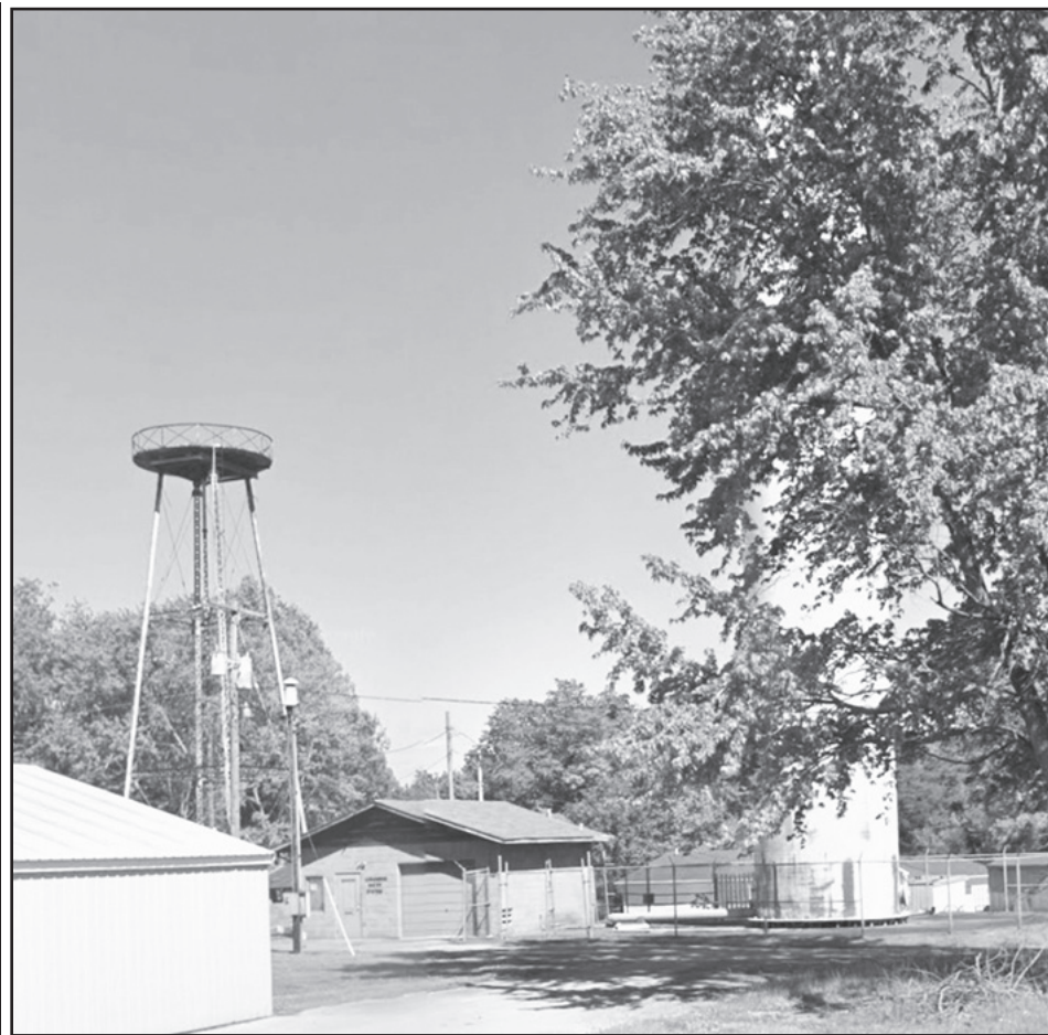
This Google maps photo shows the current Columbus, Ky. water company office. Plans for the $2.88 million grant the city has been allocated include a new water company office, high pressure pumps, and more.
