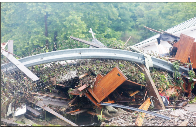
The damage from the floods has been extensive, with residences, businesses, churches, and more all taking on flood water.
