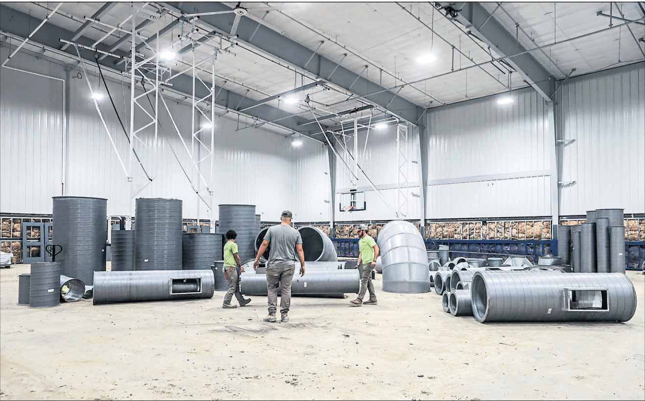
A crew moves large air ducts on the inside of the Bluegrass Fieldhouse sports complex on Thursday as construction continues.
