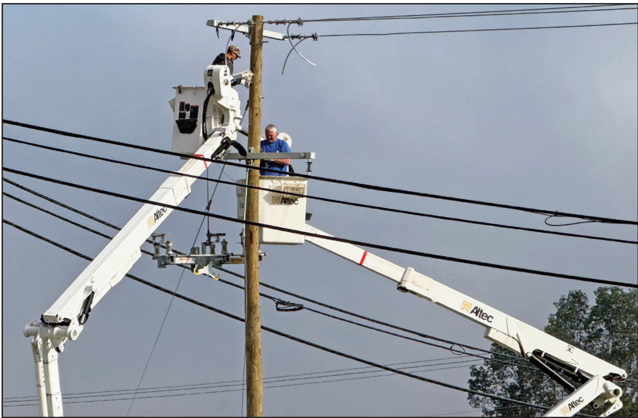
Dennis Brown/LEWIS COUNTY HERALD HIGH WIRE ACT . . . Workers with the Electric Plant Board of the City of Vanceburg perform maintenance on electric lines at Black Oak. While maintenance is an ongoing effort, crews are getting some extra work completed before winter weather sets in.
