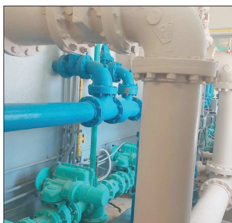
▲ PHOTO | LYNN BLEDSOE Different color pipes indicate water in different levels of treatment.
