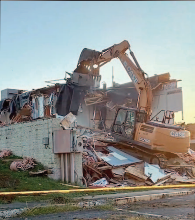
The former Crittenden Community Hospital annex, was demolished this week after being deemed structurally unsound. Crews with Superior Excavating and Trucking of Marion brought the building down Tuesday and spent the following days loading and hauling away the debris. Once the site is cleared, work will shift to grading the property, followed by seeding and spreading straw. Weather permitting, the cleanup and restoration work is expected to be completed late this week.
