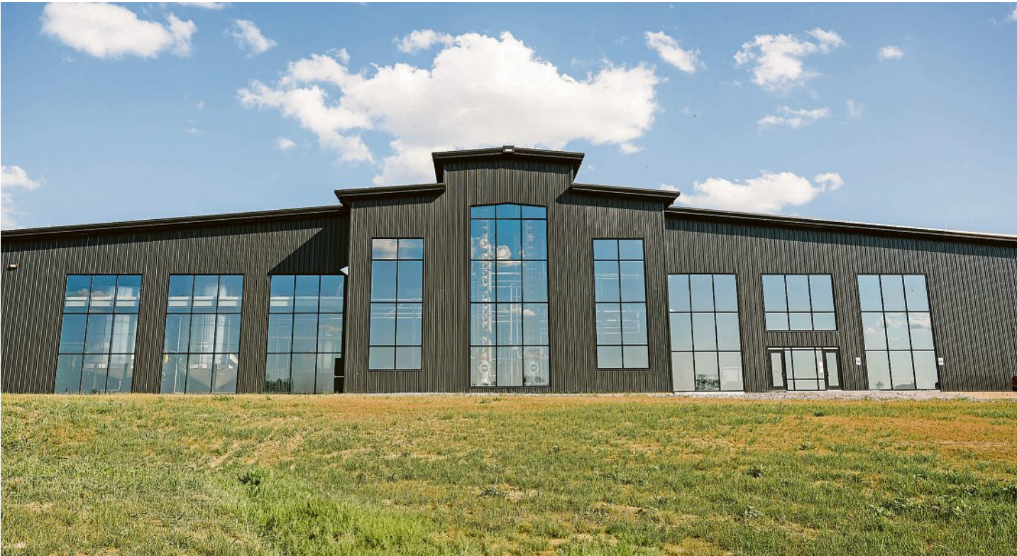
Sazerac has purchased a Lancaster facility, known as Garrard County Distilling, which sits on approximately 210 acres and includes two, 20,000-square-foot barrel warehouses. The facility opened in 2024 and closed in 2025 amid financial woes. PROVIDED BY SAZERAC
