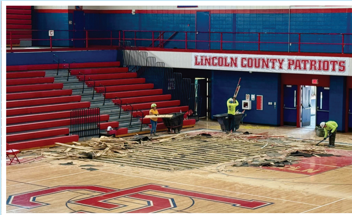
Construction crews begin removing the original gym floor at Lincoln County High School, which has served the district for nearly 50 years. The replacement is part of a larger renovation project that includes new bleachers, lighting, and facility upgrades throughout the building. (Photo submitted)
