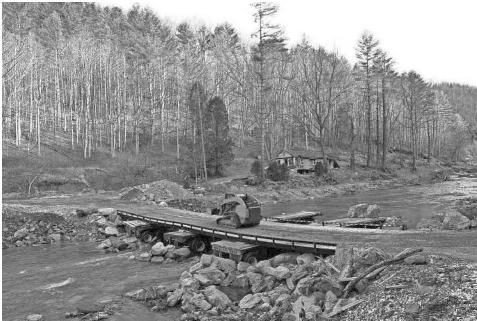
This temporary bridge at Tennessee's Poga Bridge 1 crossing was donated by Troy Henry, owner of Roadrunner Bridge in Greenville, Texas. The bridge was placed on top of semi flatbed trailers. CAITIE MCMEKIN/KNOXVILLE NEWS SENTINEL
