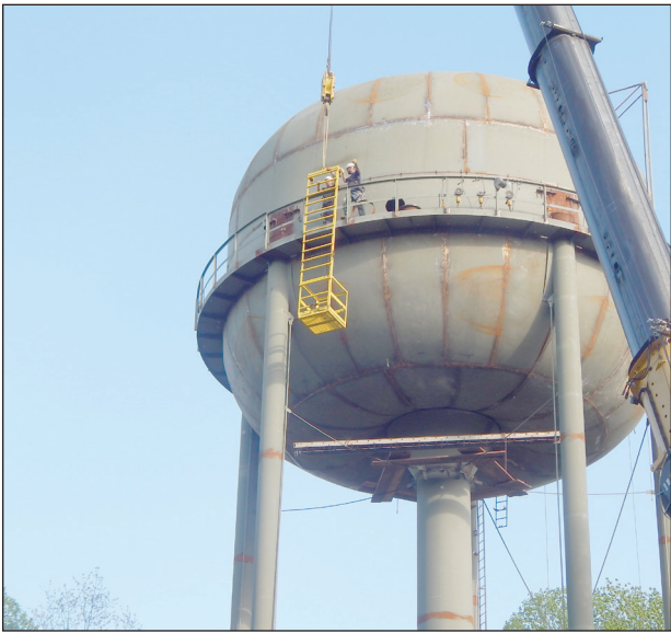
▲ PHOTO | H. D. OVERHOLT With a height of more than 100 feet, Caldwell Tank welders position the balcony cage onto the walkway by General Steel Crane operator. The cage can rotate around the bowl and will assist in completing welding operations beneath the bowl this week.
