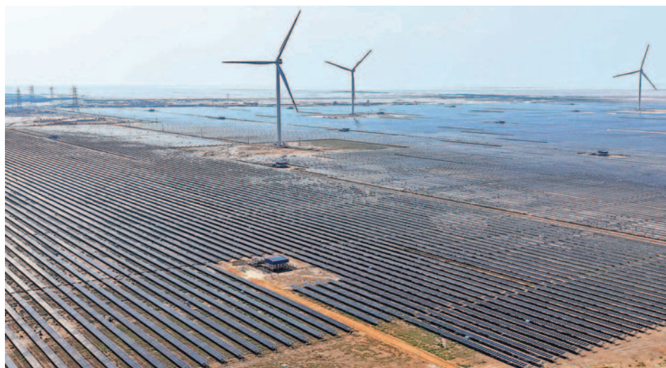
Solar panels are installed at the Adani Green Renewable Energy Plant in Khavda, in India's Gujarat state. The plant consists of some 60 million solar panels and 770 wind turbines spread over 208 square miles — almost the size of the sprawling megacity Mumbai. PUNIT PARANJPE/AFP VIA GETTY IMAGES
